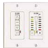
Interior Control Panel
